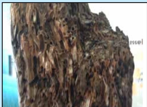
Figure 1: Part of the Busselton Jetty destroyed by Tereido worms.
